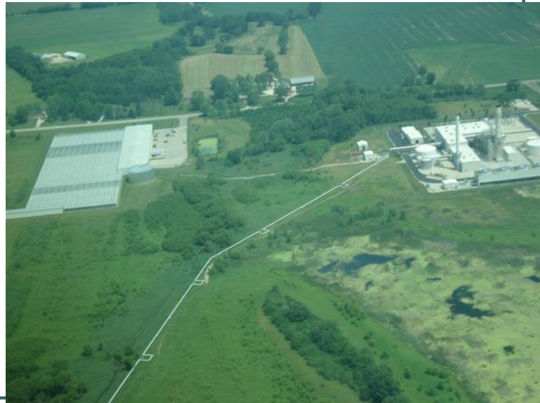
Natural gas-fired, steam co-generation plant in Whitewater, WI
