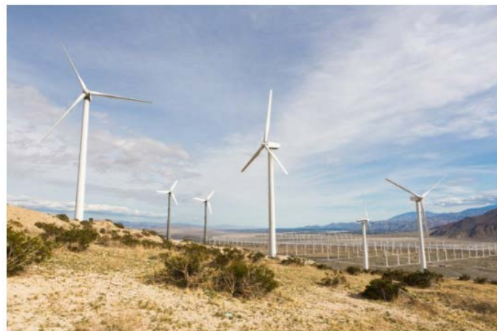
Wind turbines in the desert near Palm Springs, Calif. A recent report by Lazard, the financial advisory and management firm, found that wind power was the least costly power source. Beth Collier for The New York Times
