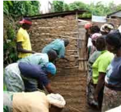
Installing small garden systems in Kenya.
